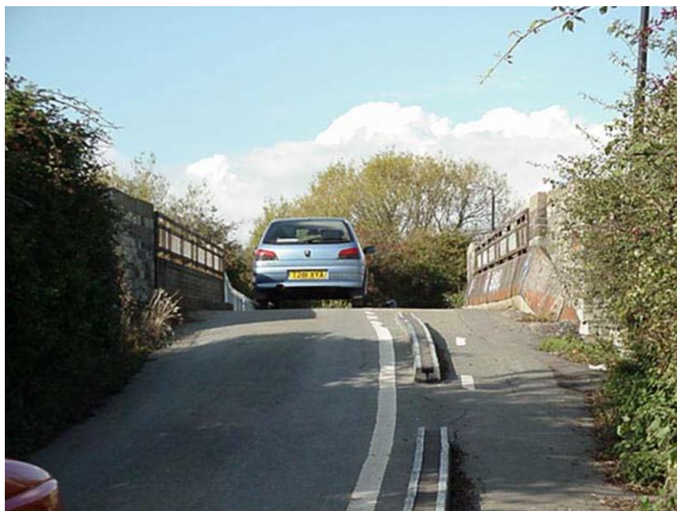
Figure 12- Segregation between footway and carriageway over an existing bridge with footway and carriageway being at the same level (Source: DfT Traffic Control System Design for All Purpose Roads Compendium of Examples)
